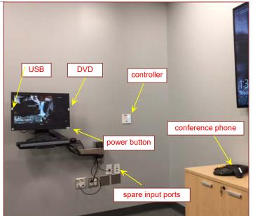
The **USB** ports are located on the left side of the computer screen. There are spare input ports below the arm mount that correspond to buttons on the wall control for additional devices such as a laptop or media players. A Polycom Soundstation is also available for conference call occasions. The phone number for use is **301-668-2604**.
