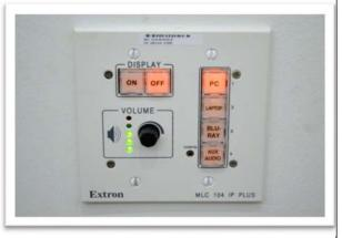
The wall or rack mounted EXTRON Control Unit controls what information is sent to the projector. The typical controls are from top to bottom: the POWER button to turn projector ON & OFF. The right buttons control which piece of equipment you want to project on the screen-COMPUTER, LAPTOP, VIDEO, ETC. The volume knob controls the sound level of the system--UP=louder, DOWN=lower. Please report blown bulbs to Help Desk ASAP. Please turn the projector OFF when not in use and before leaving room.
